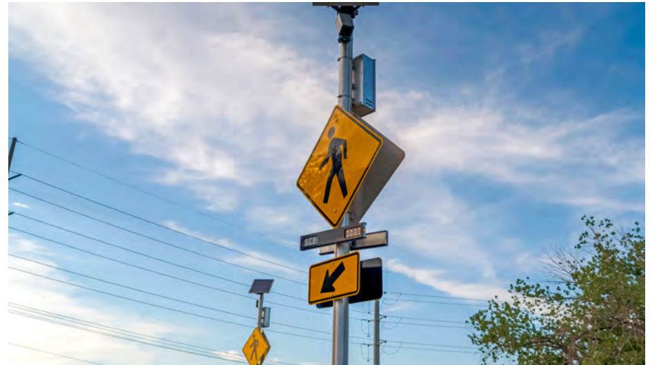
FIGURE 13. RECTANGULAR RAPID FLASHING BEACON (RRFB)
