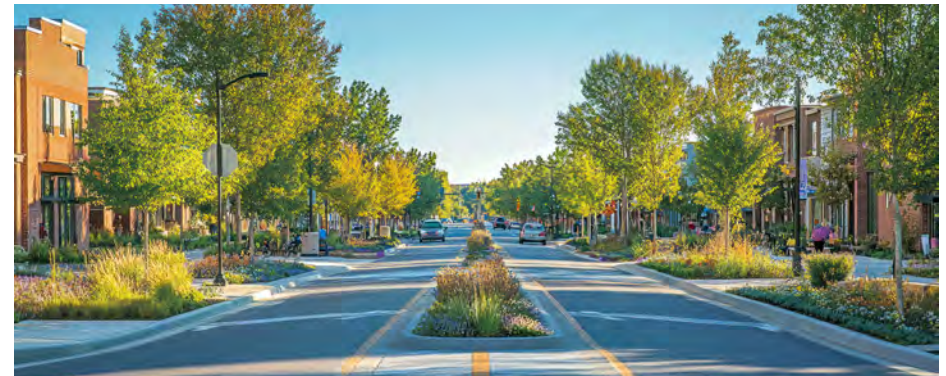
FIGURE 3. EXAMPLE OF RAISED MEDIANS
